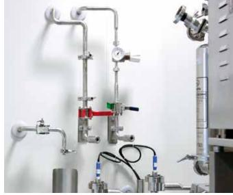
Two seals close the feedthrough according to clean-room standards: the first seal is located on the back of the CleanShut system and provides a seal between the housing and the clean room wall. The second seal is located in the inner passage of the feedthrough and seals it off. This design thus makes using additional sealants unnecessary.
